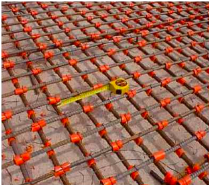
Standard requirement for isolation of steel which is time consuming and not always 100% effective
