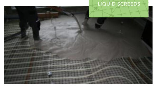
In the past welded wire steel reinforcement provided crack control in screeds. Now Orlimex offer an easy to use Basalt Fibre Reinforced Polymer (BFRP) mesh reinforcement - ORLITECH.
