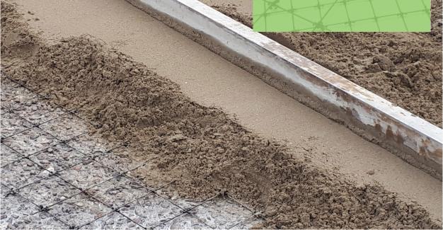
In the past welded wire steel reinforcement provided crack control in screeds. Now Orlimex offer an easy to use Basalt Fibre Reinforced Polymer (BFRP) mesh reinforcement - ORLITECH.
