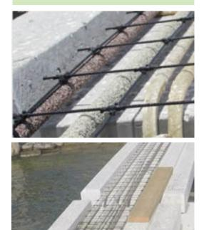
The use of seawater in the concrete mix allows the production of a more sustainable concrete structure by eliminating the use of freshwater, a scarce resource. The concrete dock was constructed using precast elements of piles, pile caps and slabs. The piles and pile caps were reinforced with FRP rebar in place of steel rebar and the slabs were reinforced with basalt fibre reinforced polymer bars and mesh. This structure was designed to withstand wind and wave loads of a category five hurricane.
