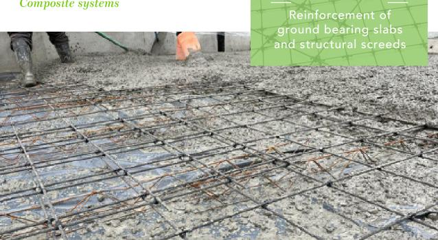
In the past welded wire steel reinforcement provided crack control in non-structural ground bearing slabs and structural screeds. Now Orlimex can offer an easy to use Basalt Fibre Reinforced Polymer (BFRP) mesh reinforcement - ORLITECH®
